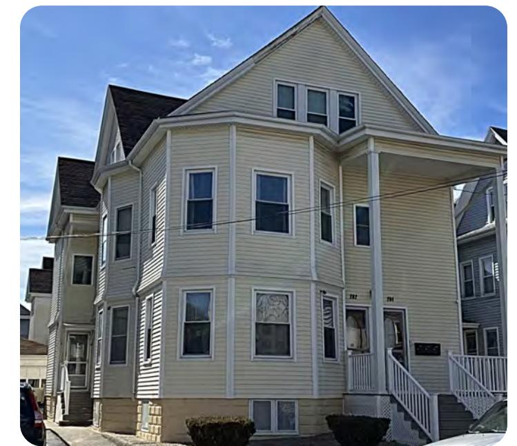
In the early 1990s, Joao and Julia Temoteo moved to the U.S. from Portugal with their two children and purchased their forever home — a three-level multifamily property in New Bedford, Massachusetts, constructed in 1915. Through the Mass Save Programs, they made air sealing, insulation, and ventilation improvements as well as wiring upgrades — all at no cost. Less than a year after the project was completed, the family can now comfortably use all three rooms of their third-floor apartment. In addition to the up-front cost savings, the family is projected to see approximately $1,000 in annual energy savings.
