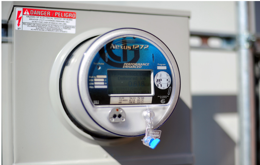
Photo: A “smart meter” capable of Advanced Metering Functionality
