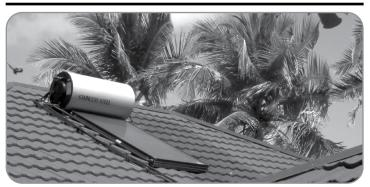
The heated fluid then goes to a storage tank where it heats water. The hot water may then be piped to a faucet or showerhead. Most solar water heaters that operate in winter use a heat transfer fluid, similar to antifreeze, that will not freeze when the weather turns cold.
