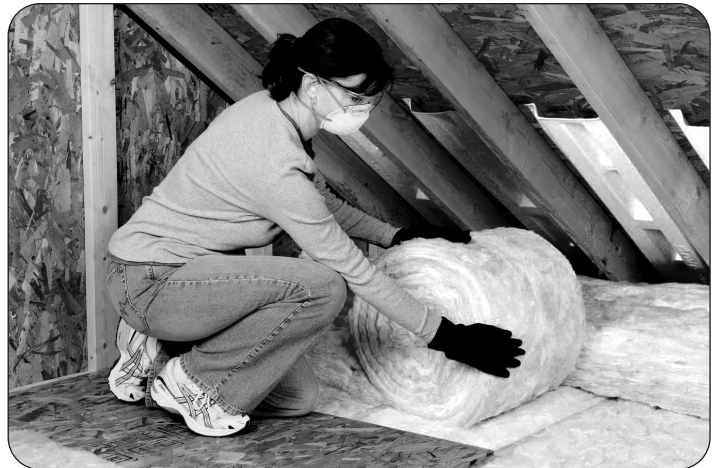
Image courtesy of Owens Corning
