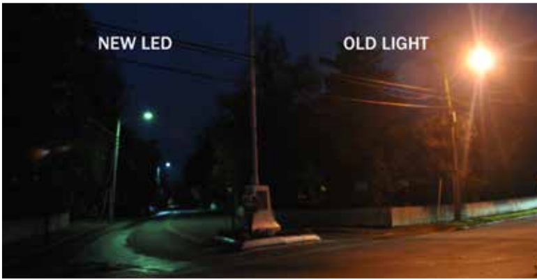
Edgartown before and after LED streetlight installation
