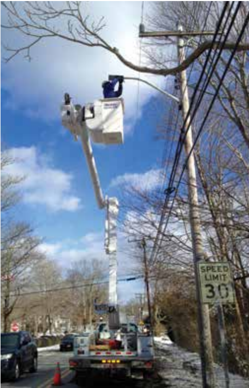
LED streetlight installation in Brewster
