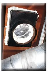
indoor environment and lowering energy bills. In typical homes, air leaks are often found at cracks, small holes, and penetrations for plumbing, wiring, lighting, and duct work.
