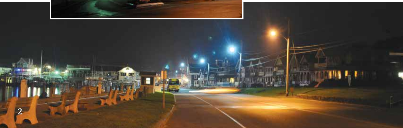
Oak Bluffs LED streetlight installation
