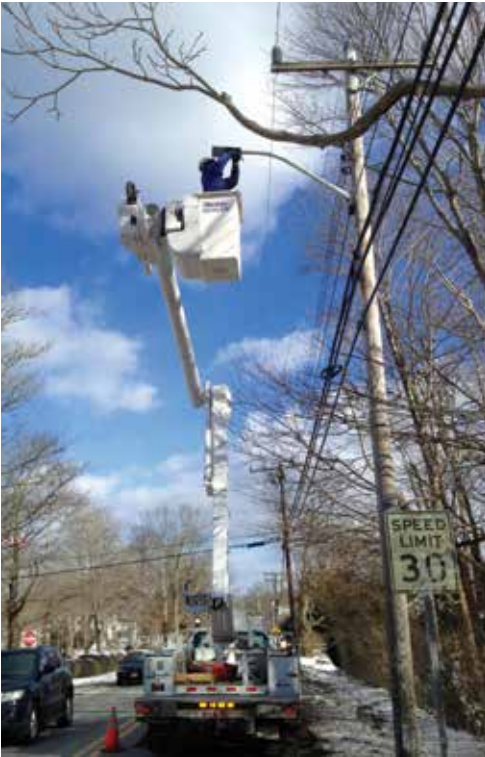
LED streetlight installation in Brewster
