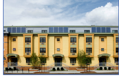
Trolley Square Development, courtesy of MassHousing
