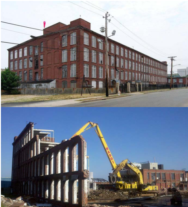
Tillotson Complex – Mill #1 Built in 1887, Demolished in 2011. (total of 400,000 sq ft. razed in complex.)
