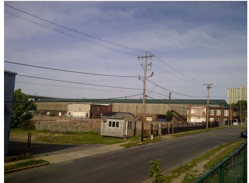
Former Mill #1 – May 18, 2012 (Green roofed building is TPI R&D facility for wind turbine blade co.)
